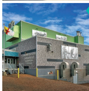
Accutech Engineering Inc. was presented with an Award of Excellence and the prestigious Engineering a Better Canada Award for the Arvilgruaq Ilinniavik School in Kugaaruk, Nunavut.
