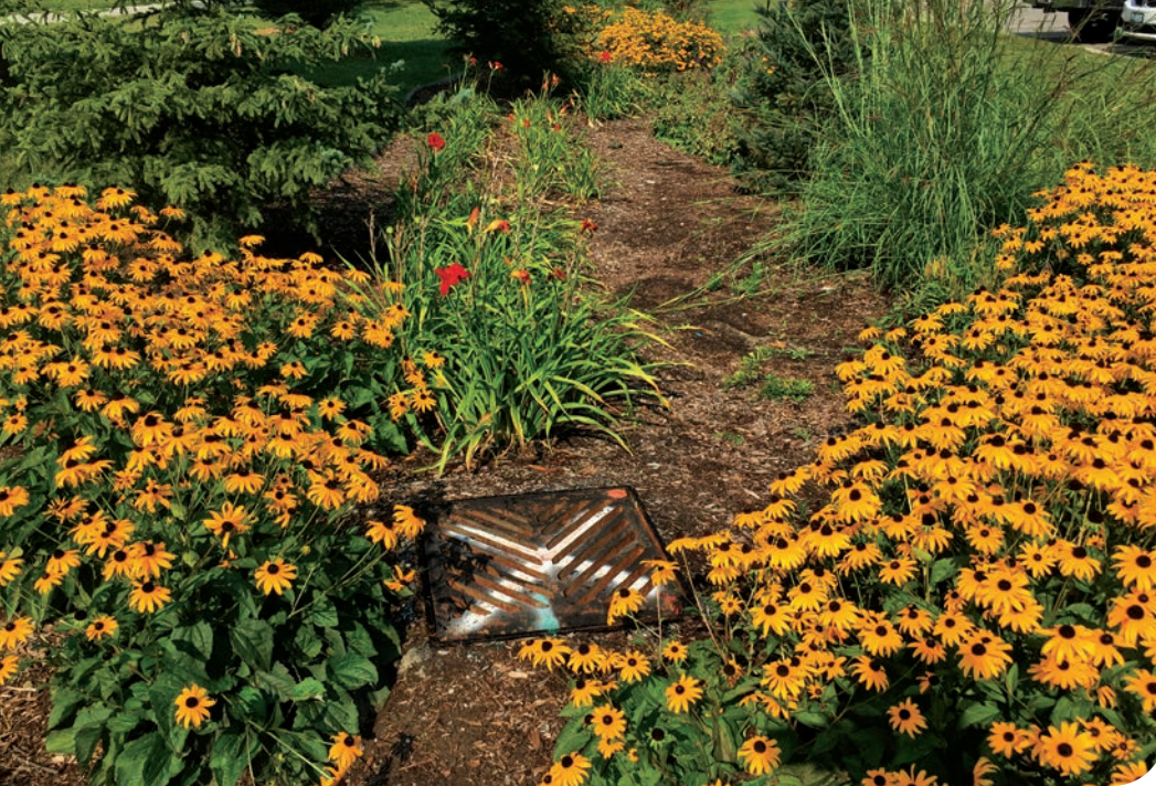
A bioswale is a type of low-impact development used by LSRCA to effectively manage stormwater and protect wetlands. Photo: LSRCA
